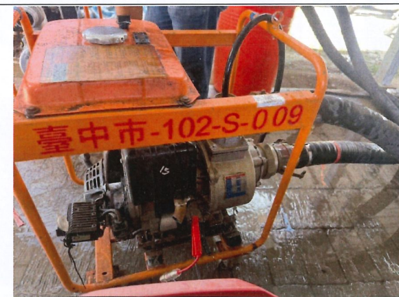
102-S009-07-抽水機試車前
