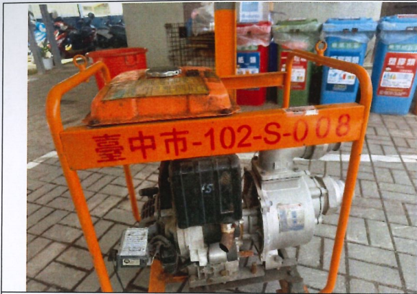
102-S008-01-抽水機檢查前
