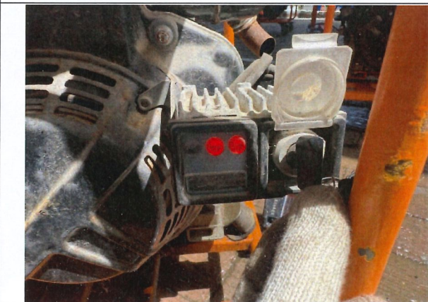
102-S007-07-抽水機試車前
